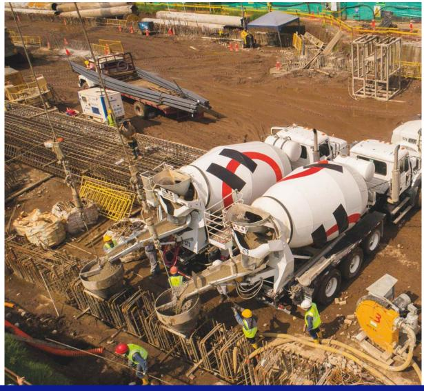
Armed and concrete placement through tremie pipe
